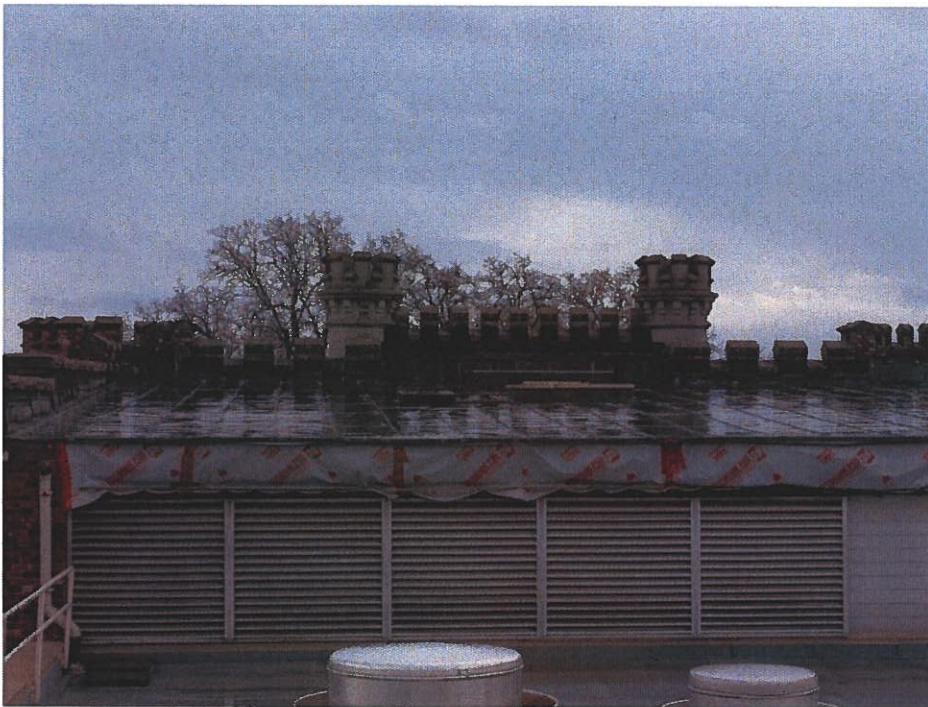
Section of roof to receive a new roof
